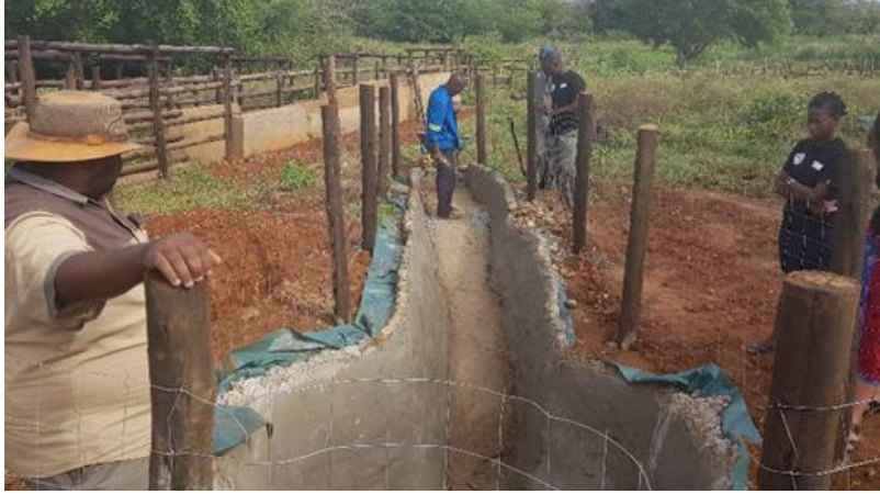
The Mboza dip tank being waterproofed before use
